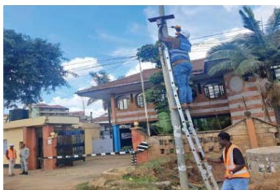
1. Engineers install an air quality monitoring device along a major traffic corridor in Kiambu County as part of the county's clean energy and air quality monitoring initiative.
