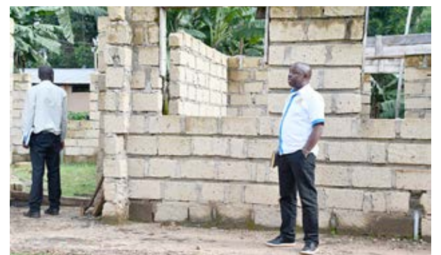
CDE, PHILIP CHIRCHIR, Kisii County inspect the stability and security of the structure in one of the schools in Nyamache Sub county, Kisii.
