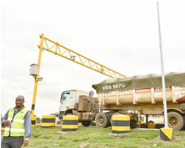
A long-distance cargo truck passes through one of the recently installed high-motion sensors to detect load weight and ensure compliance with strictly enforced load weight for both local and transit transporters
